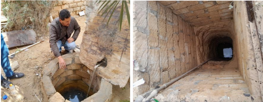
Figure 5: Wells photographs illustrating spatial variations in groundwater depth, ranging from less than 1 m below ground surface in the northwestern of the city (near Ajdabiya Municipality) to more than 6 m in the eastern sector (Damascus Neighborhood).
